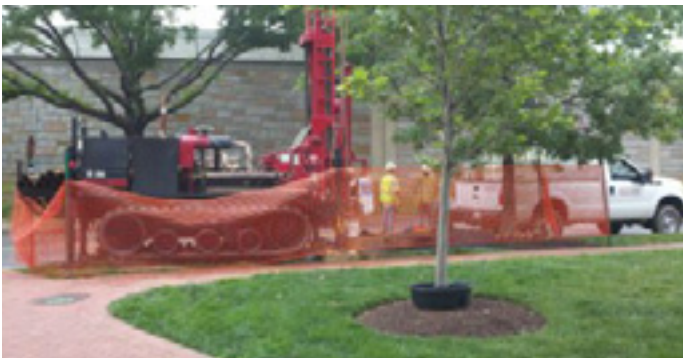
The geotechnical boring team at work along Virginia Avenue.
