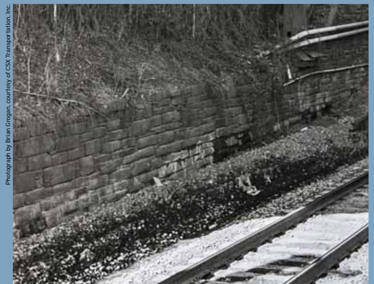
Retaining walls constructed of Seneca sandstone, shown here in 2014, extended from the east portal to protect the below-grade track. The 1872 retaining walls exhibit an ashlar pattern with irregular courses using stones of varying sizes.
