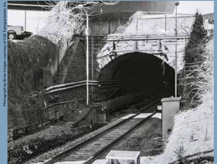
The east portal, shown here in 2014, was constructed from 1870-1872. The portal was a segmental arch made of Potomac Bluestone.
