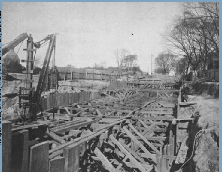
Timber cribbing for the brick arch of the 1904-1906 construction. (1904)
