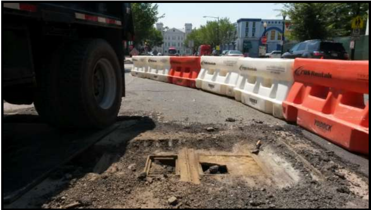
1892 streetcar slot and wheel rail and access panel frame (VAT-2015-HB-001) on 8th Street SE, with the Navy Yard gate in the center background and the Navy Yard Car Barn (blue brick building) on the right background, looking south
