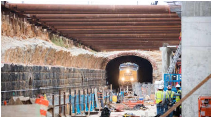
The two new Virginia Avenue tunnels will converge at the new structure's west end. A 300-foot portion of the old tunnel was demolished to accommodate work on the first new tunnel.
