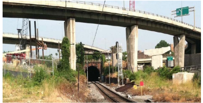
A view of the east portal of the Tunnel
