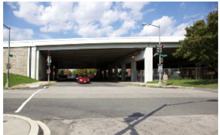
7th Street intersection at Virginia Avenue SE: north-south crossing will remain open throughout construction
