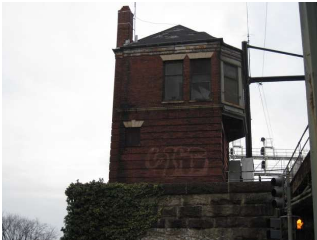
Figure 9. West Elevation, Control Point Virginia Tower.
