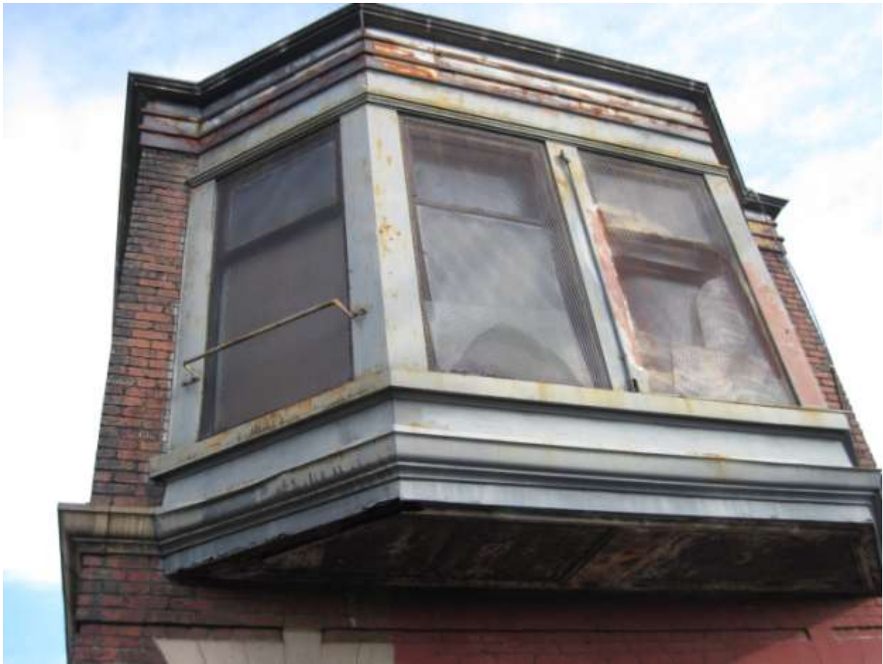
Figure 6. Bay Window, South Elevation, Control Point Virginia Tower.
