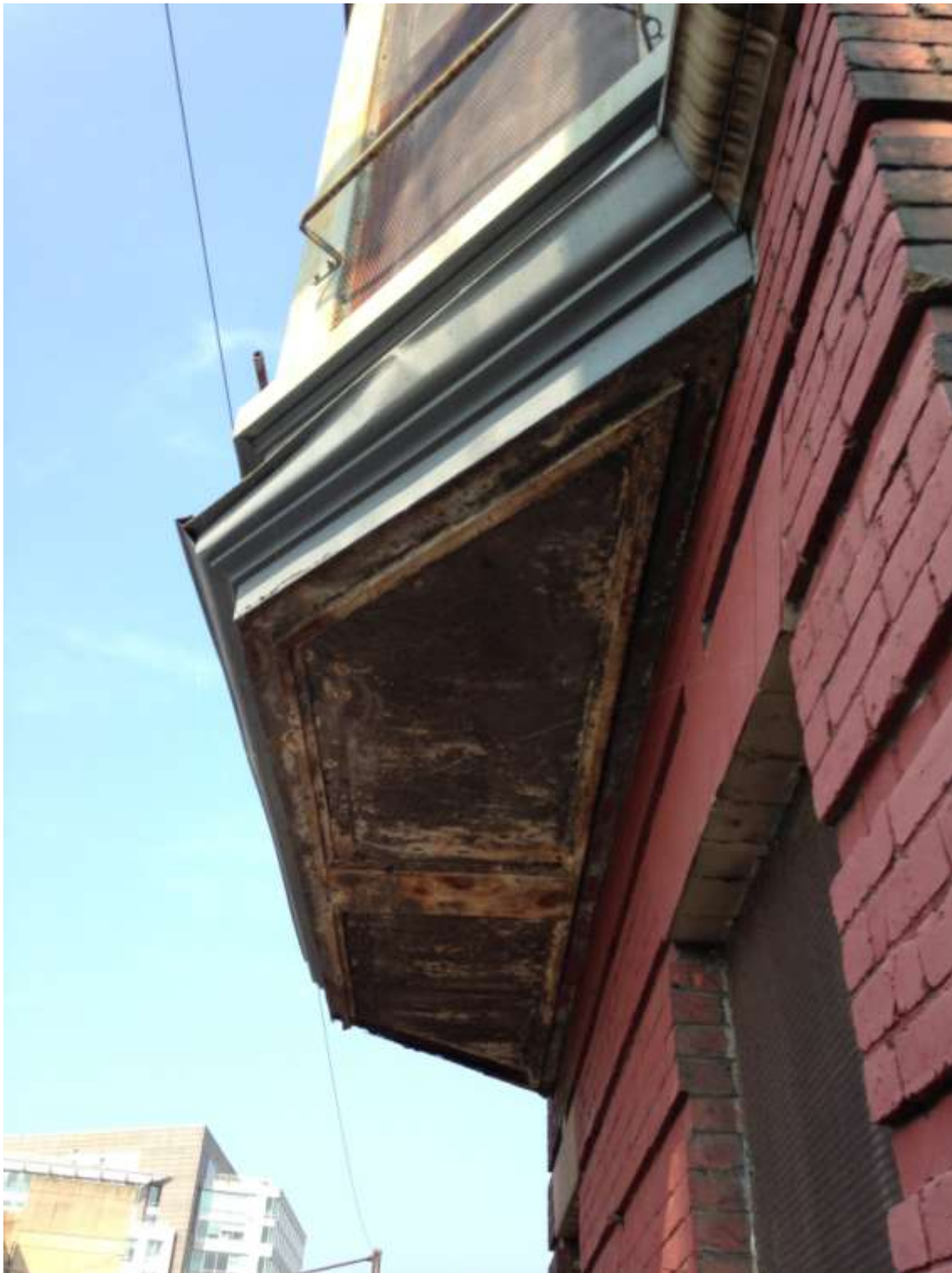
Figure 7. Bay Window Soffit, South Elevation, Control Point Virginia Tower.
