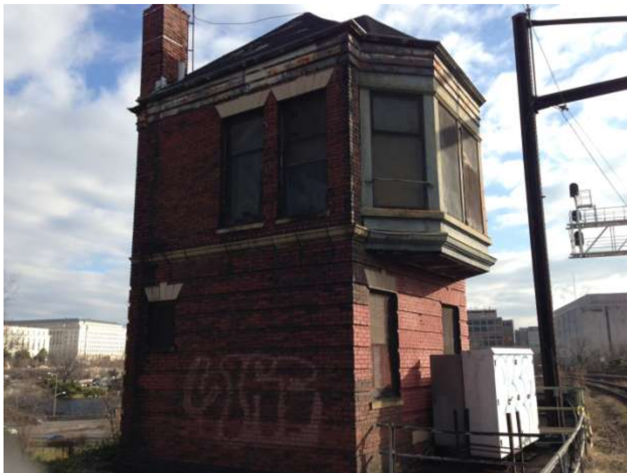
Figure 5. West and South Elevations, Control Point Virginia Tower.
