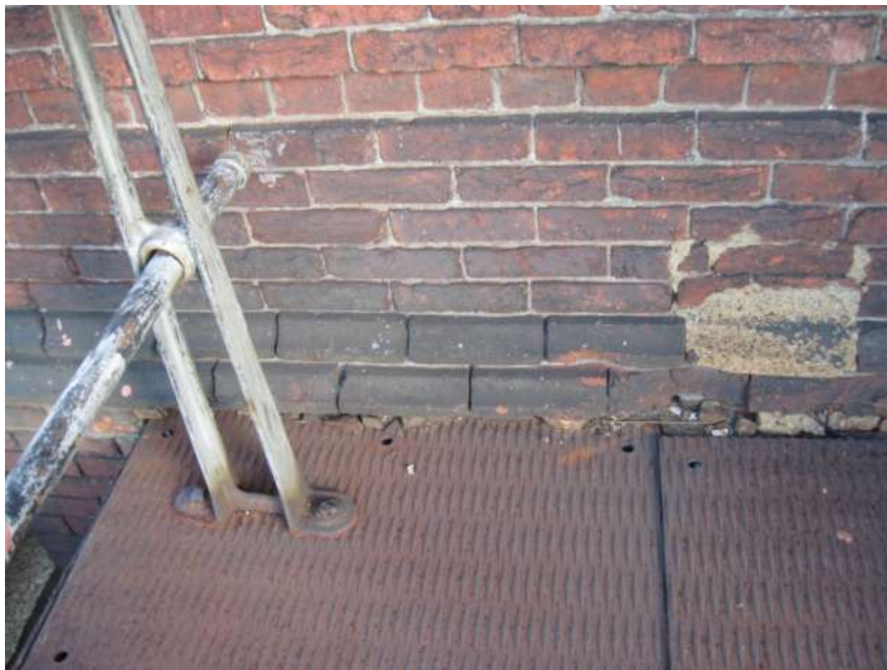
Figure 4. Water table consisting of two rows of red concave plinth bricks, Control Point Virginia Tower.
