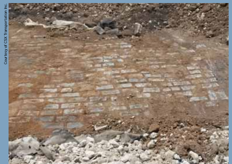
Blue scoria brick segment prior to removal.
