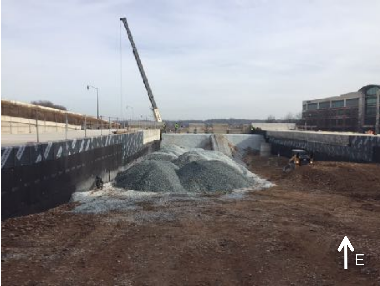
Backfilling Between the Two Tunnels
