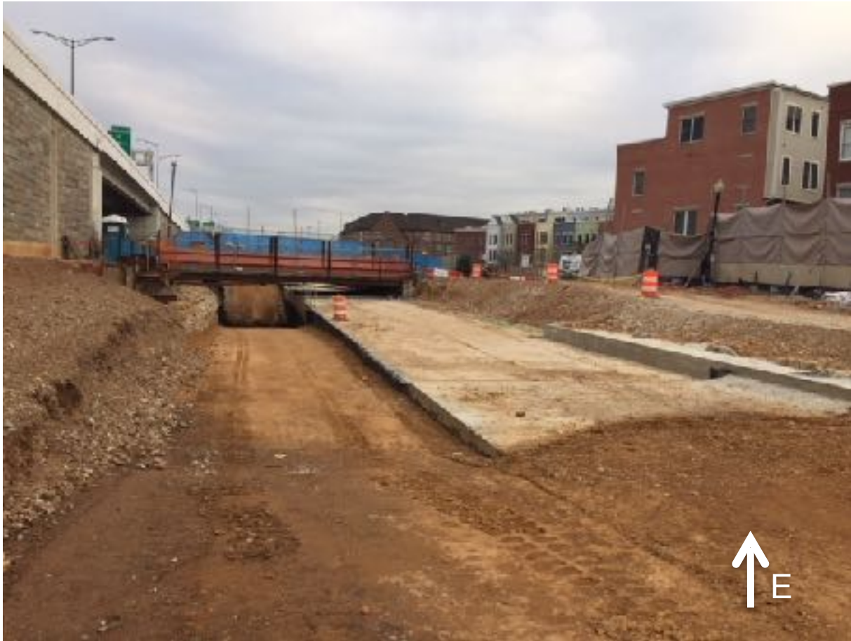
Preparing for Waterproofing
