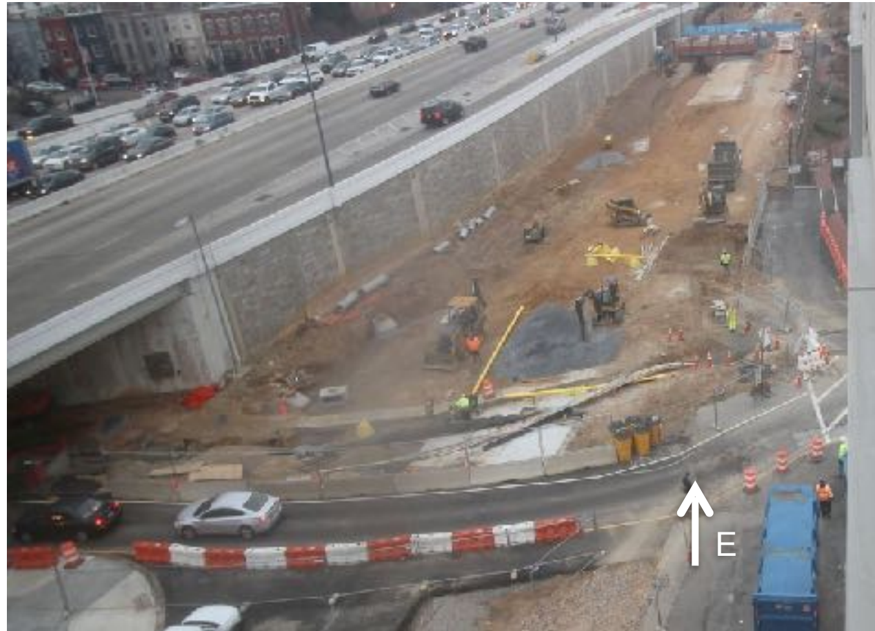
Gas Line Restoration
