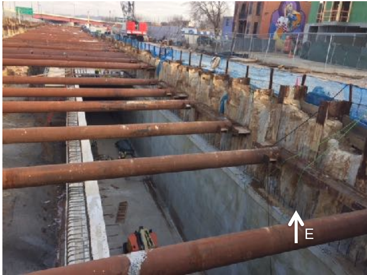
Tunnel Wall Construction
