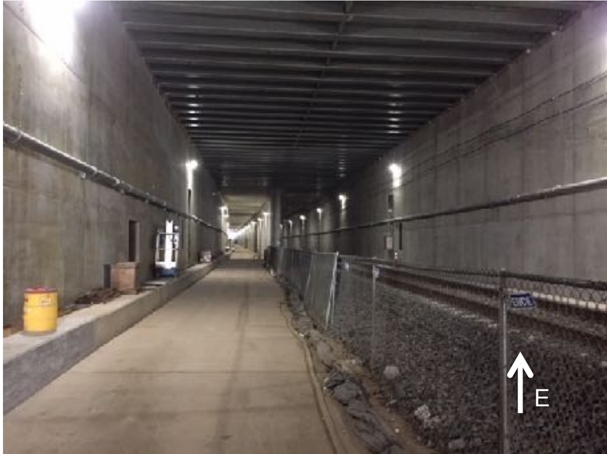
Inside the Phase II Tunnel
