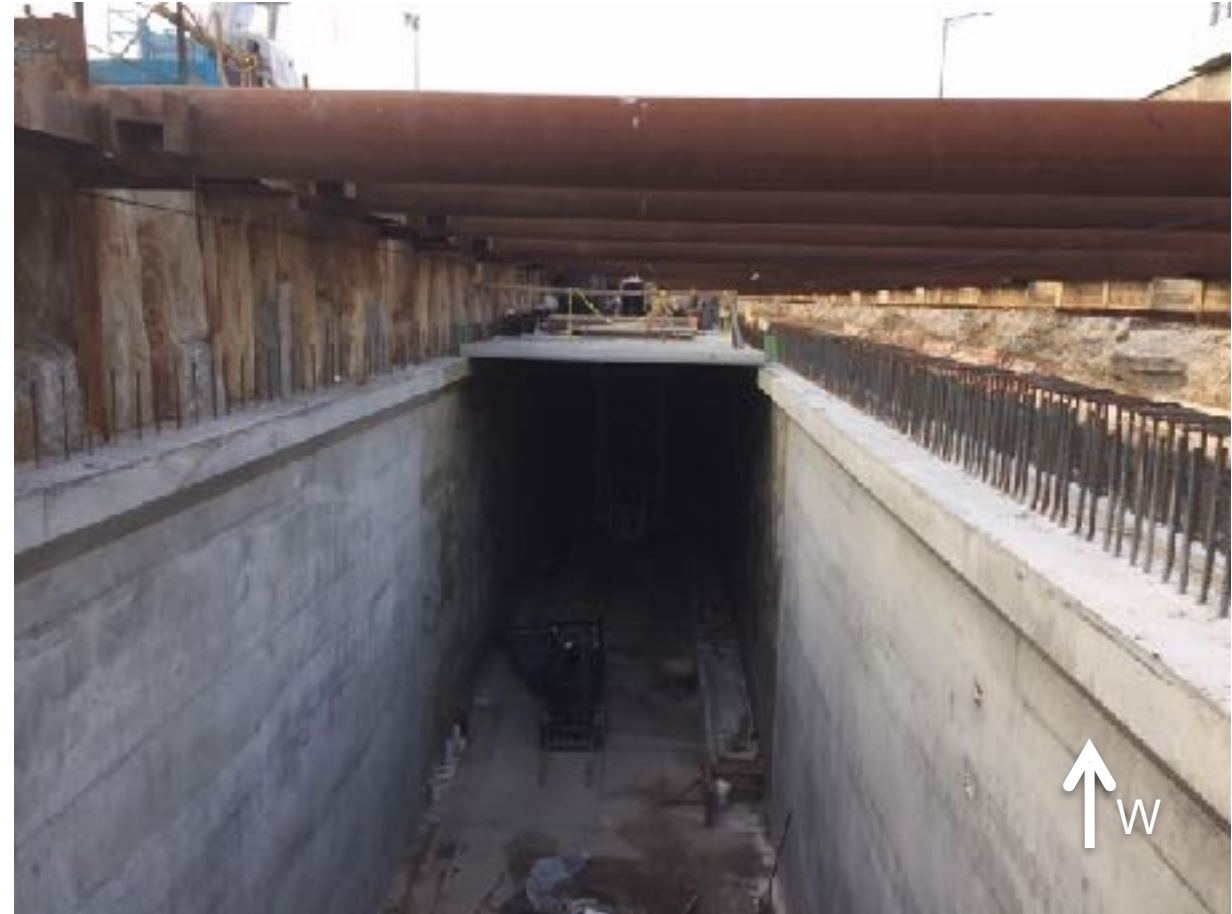
Installing Roof Panels
