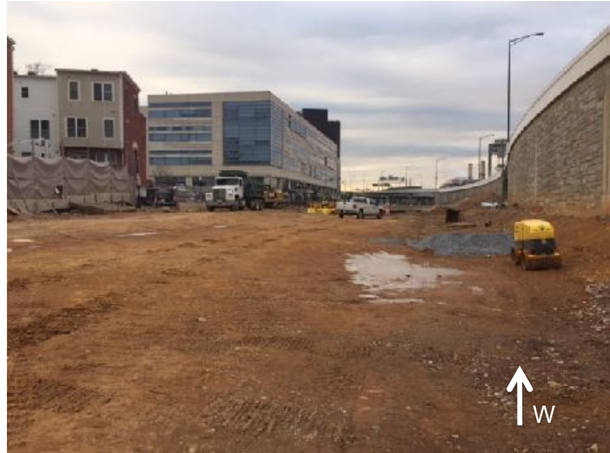
Backfilling and Compacting
