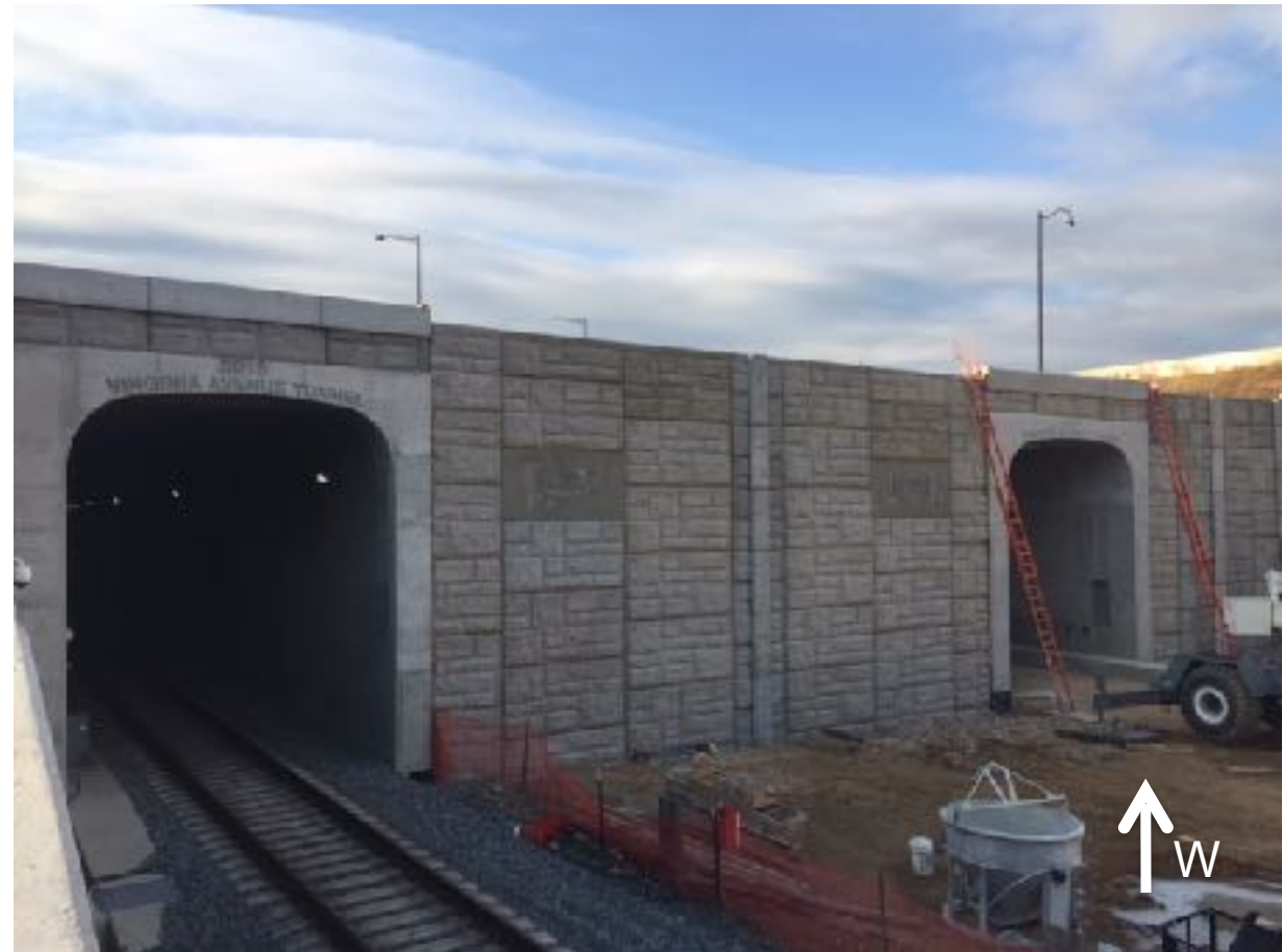
North Portal Wall
