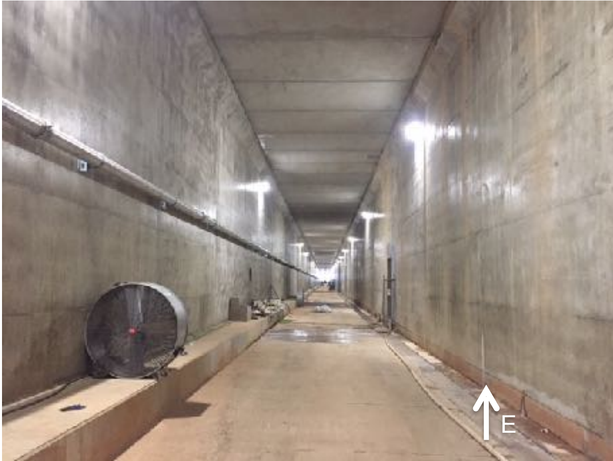
Inside the Phase II Tunnel
