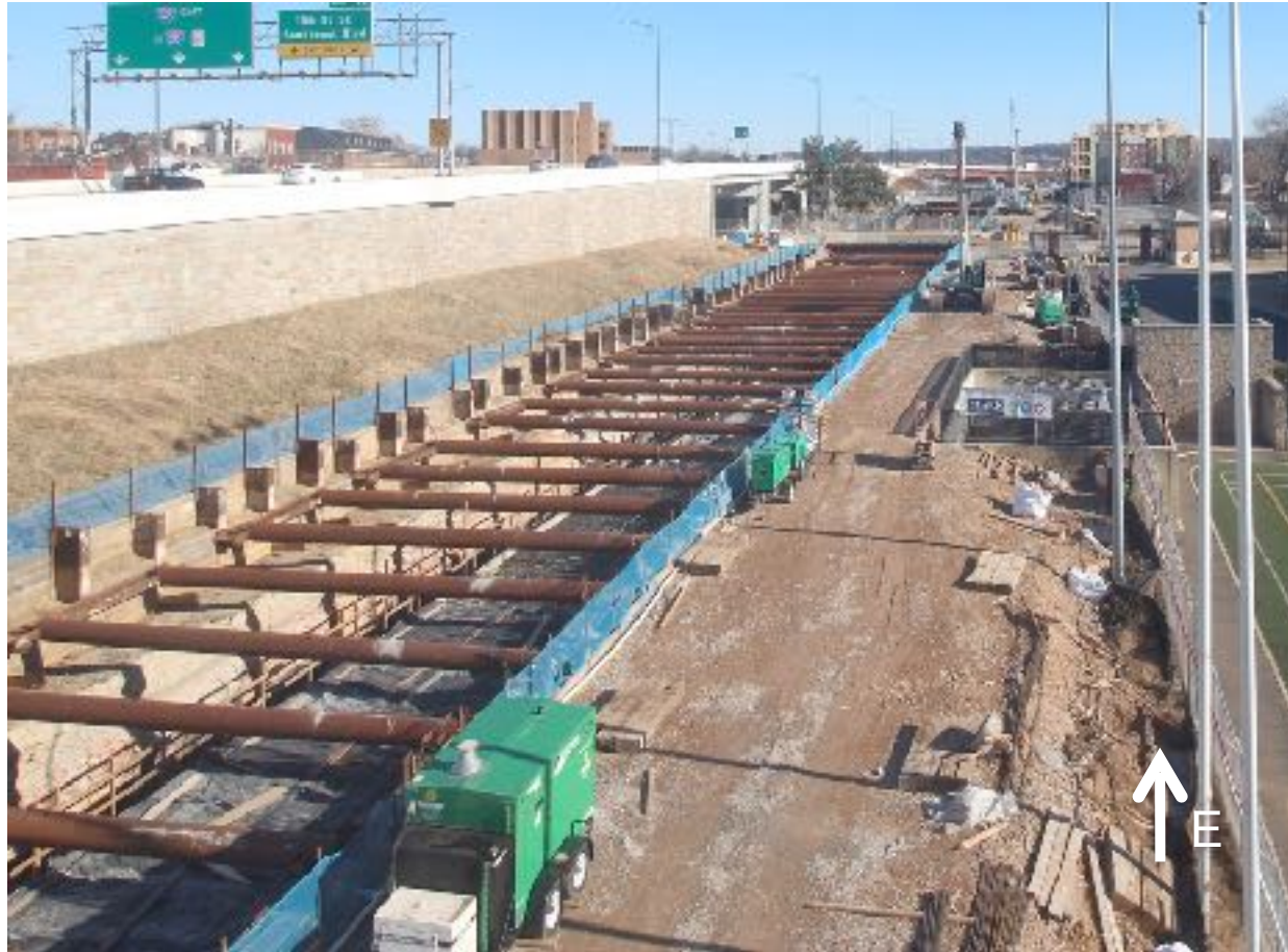
Preparing for Roof Pours
