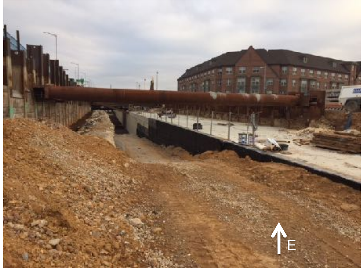
Waterproofing and Backfilling
