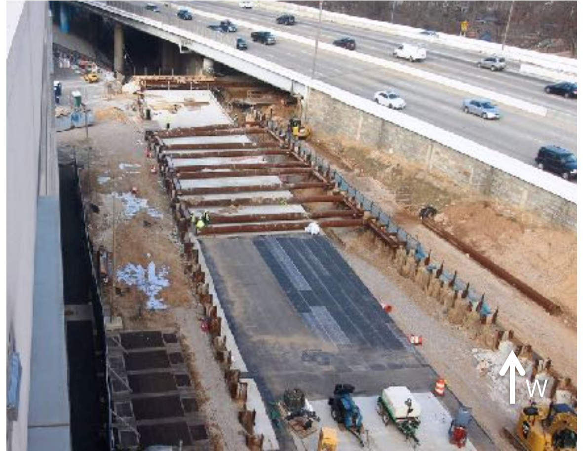
Installing waterproofing and Backfilling
