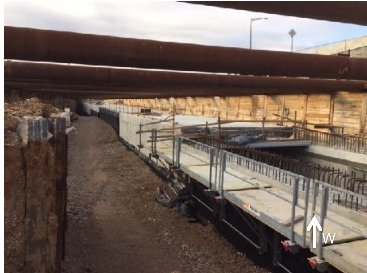
Waterproofing and Backfilling
