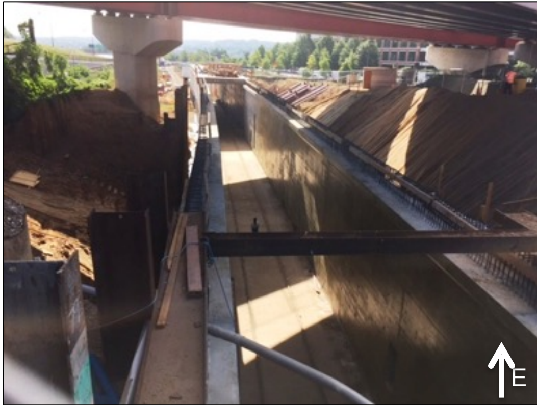
Tunnel Wall Construction
