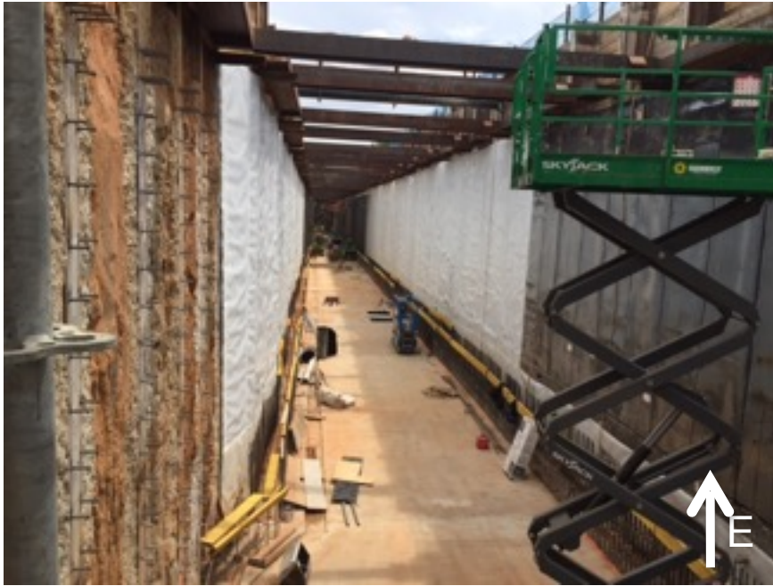
Waterproofing Installation
