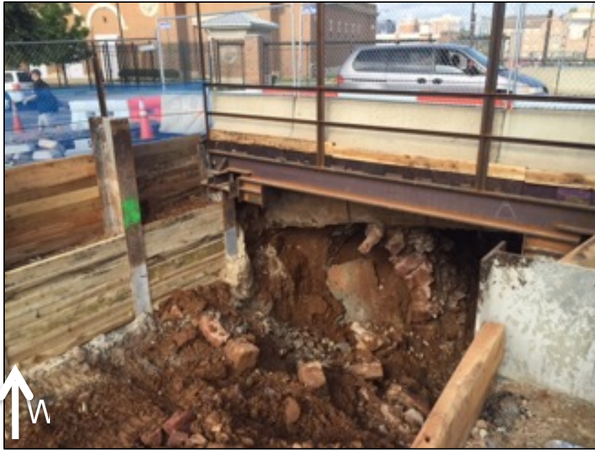
7th St. - Old Tunnel Arch
