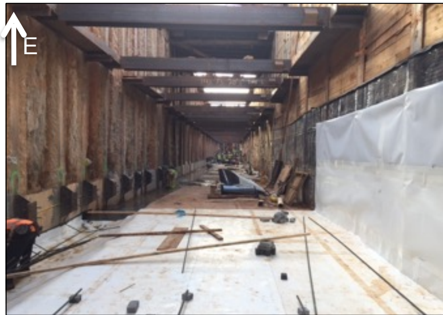
Tunnel Invert Construction
