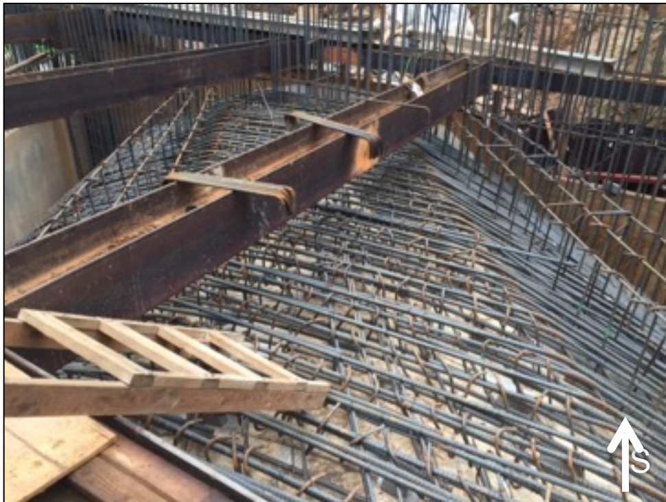
Forming the Spandrel Arch
