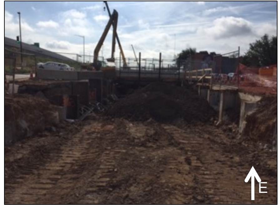
Final Phase 1 SOE Piles Drilled
