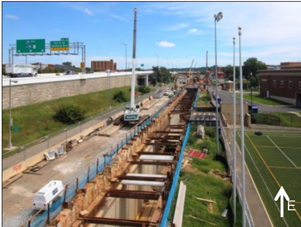
5th/6th-7th Tunnel Construction
