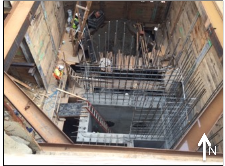
6th St. Siphon South Structure
