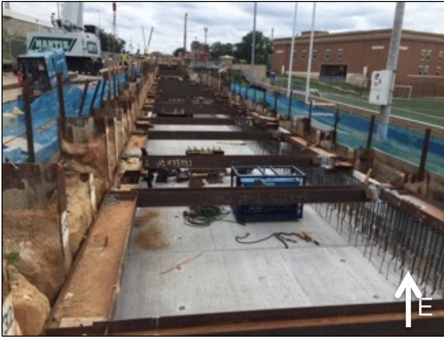
Precast Roof Soffit Panels
