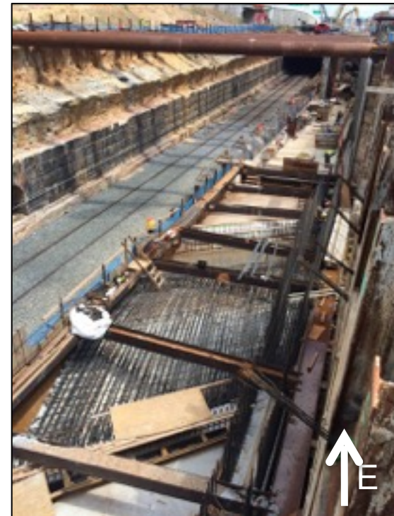
Forming the Spandrel Arch
