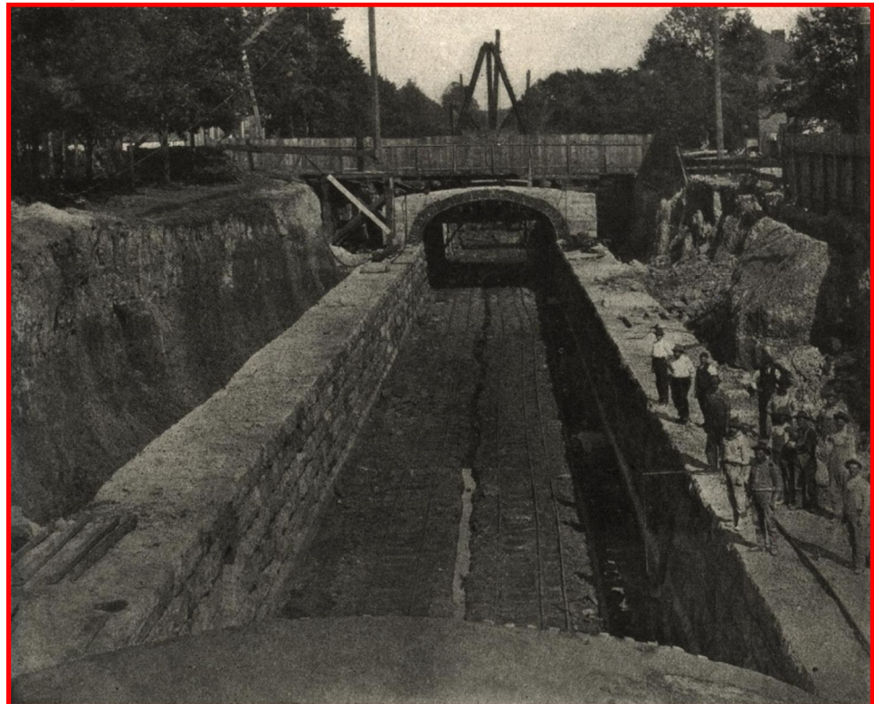
Virginia Avenue Tunnel Construction
